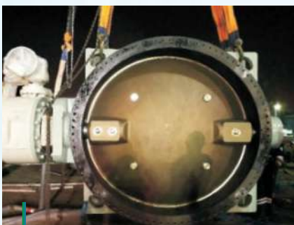
Butterfly Valve Replacement
