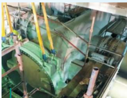
Butterfly Valve Installation
