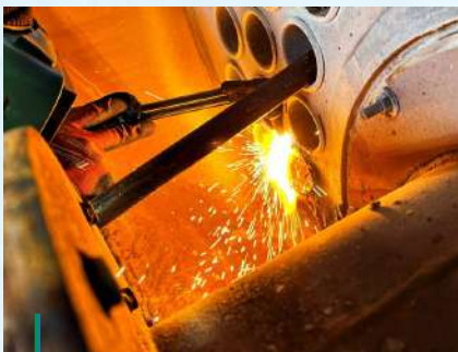
Boiler Tube Edge Preparation
