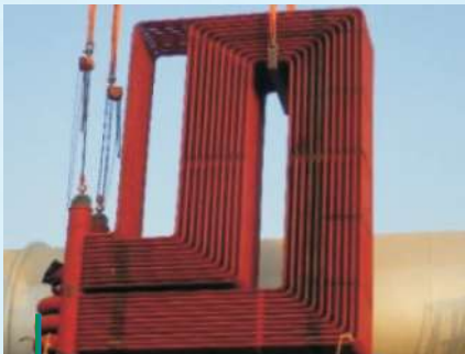
Boiler Super Heater Installation
