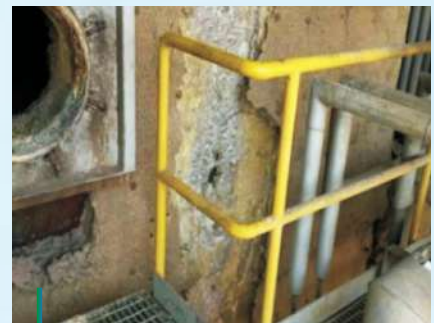
Boiler Insulation Repairing
