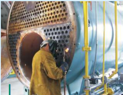
Boiler Tubes Cutting & Edge Preparation
