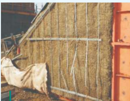
Gasduct & Insulation Work
