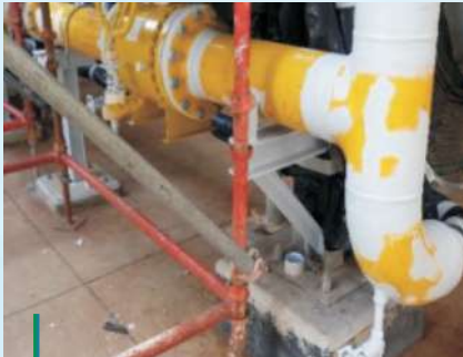
Main Cooling Water Debris Filter Cleaning
